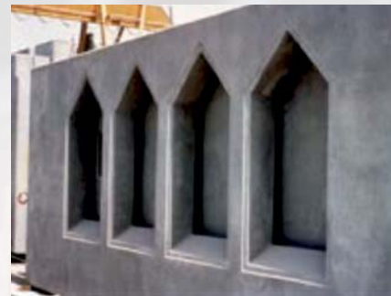
Massive semi-finished wall in the project of schools building
